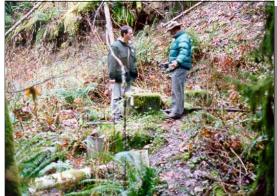
Carl Garrison of Garrison Engineering evaluates the Glacier Springs collection structure.
